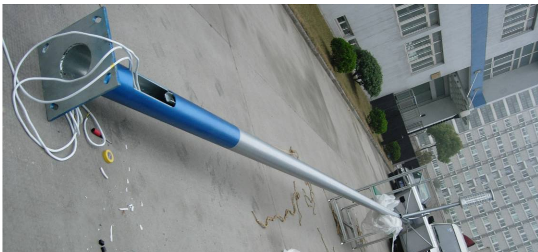
Connect the solar panel and the controller, and put the wire into the pole through the T frame, and fixed the T frame to the pole tightly, and finish installation..
