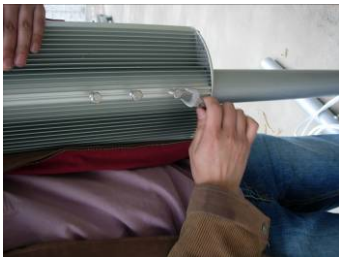
Install the lamp to the arm and screw tightly
