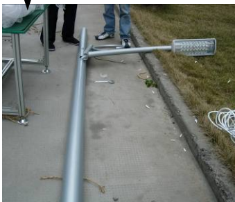
Install the arm to the pole and screw tightly
