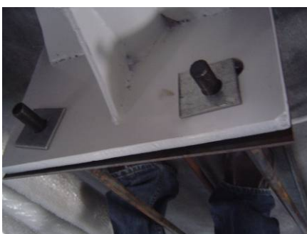
Lifting the pole with crane and put it on the underground work.
