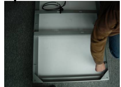
Fixed the solar panel on the frame
