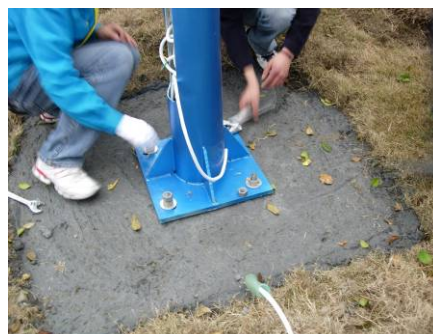
Screw down two nuts on each bolt.
